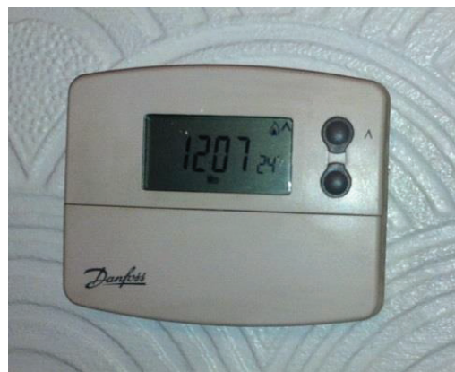
Figure 1(b). Thermostat control
