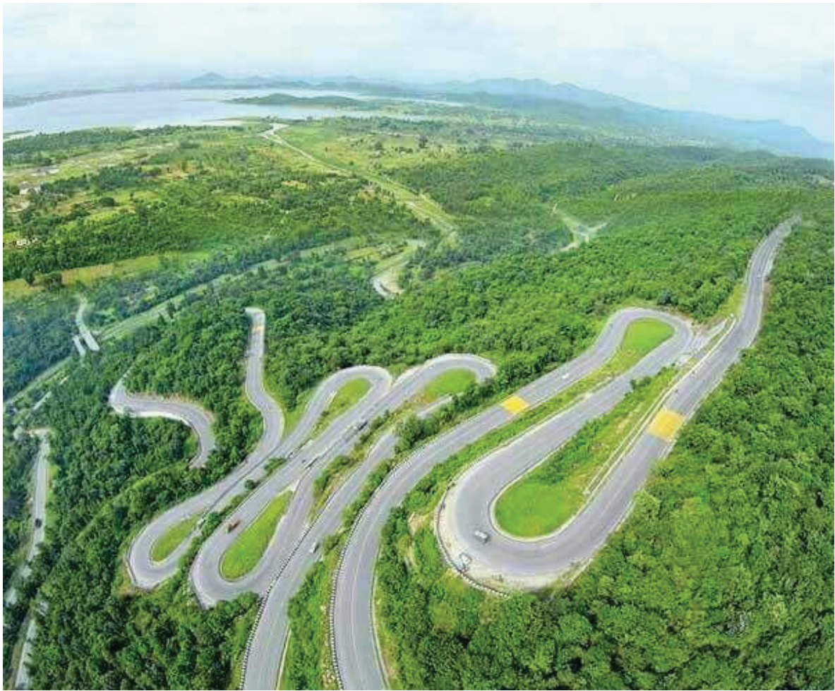
Figure 1. Switchbacks are often designed into steep terrain to make an ascent easier. Often seen in hiking trails or roadways, such as this image from Patraru, Jharkhand, India. ( https://commons.wikimedia.org/w/index.php?curid=59833771 )
