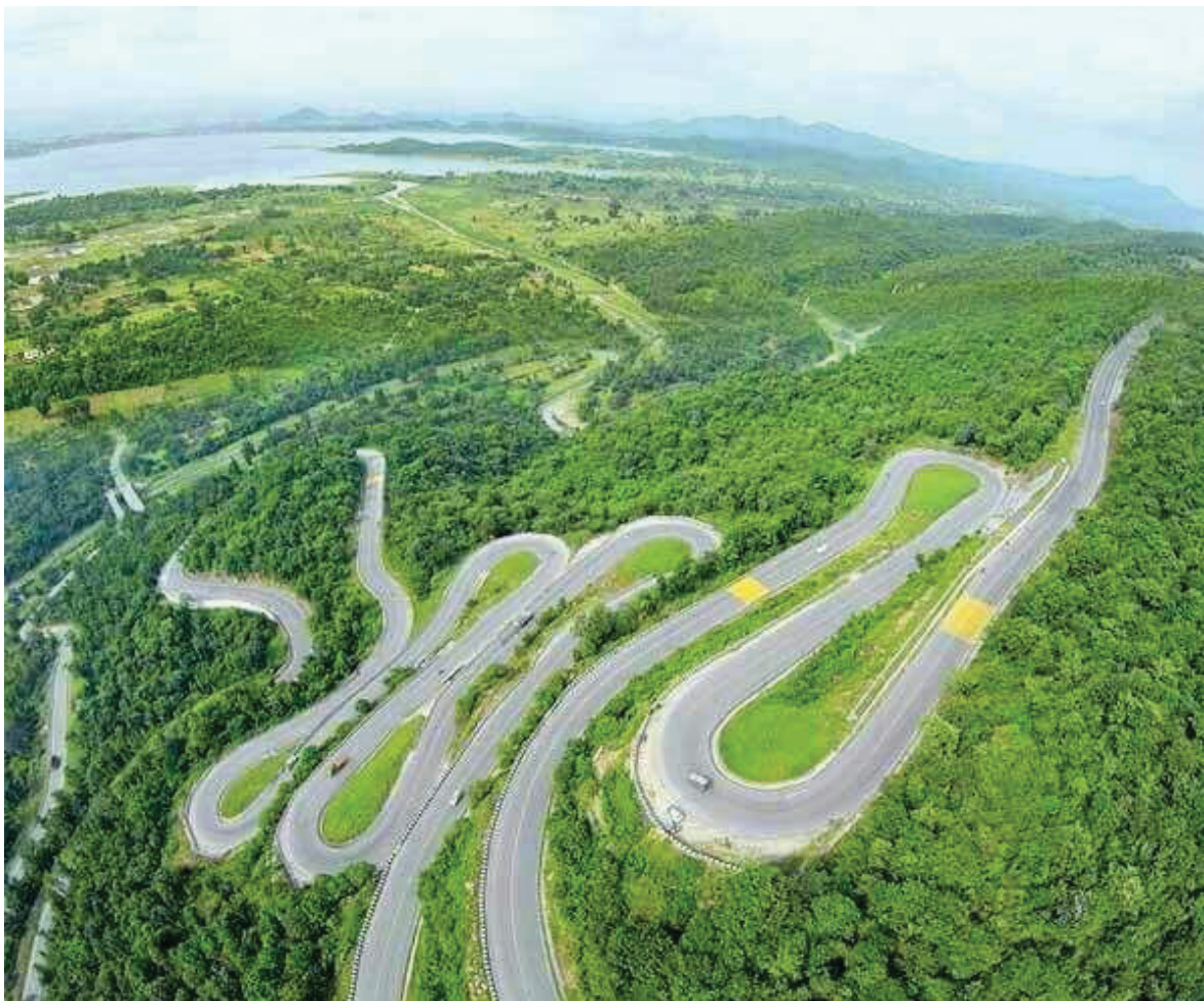
Figure 1. Switchbacks are often designed into steep terrain to make an ascent easier. Often seen in hiking trails or roadways, such as this image from Patratu, Jharkhand, India. ( https://commons.wikimedia.org/w/index.php?curid=59833771 )
